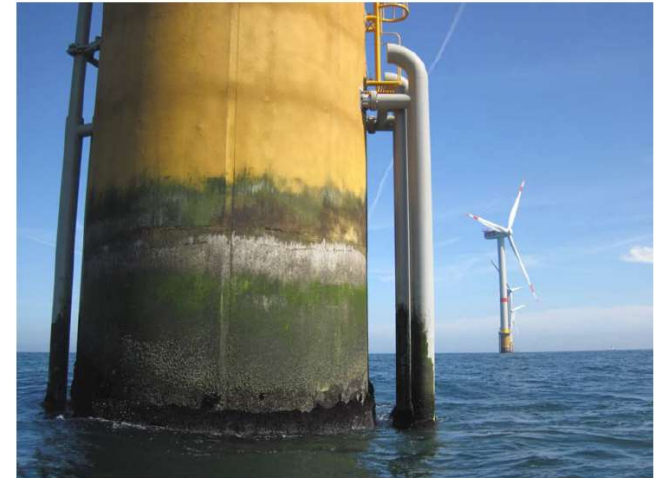
Figure 1. Concrete C-Power GBF foundation (D5) with epifouling in the eulitoral and splash zone (situation early 2011).
